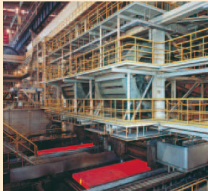
連続铸造機/Continuous Casting machine
